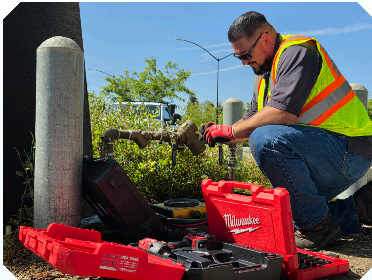
Backflow Prevention Assembly Testing - A Certified Cross-Connection Specialist repairing a City-owned backflow assembly.
