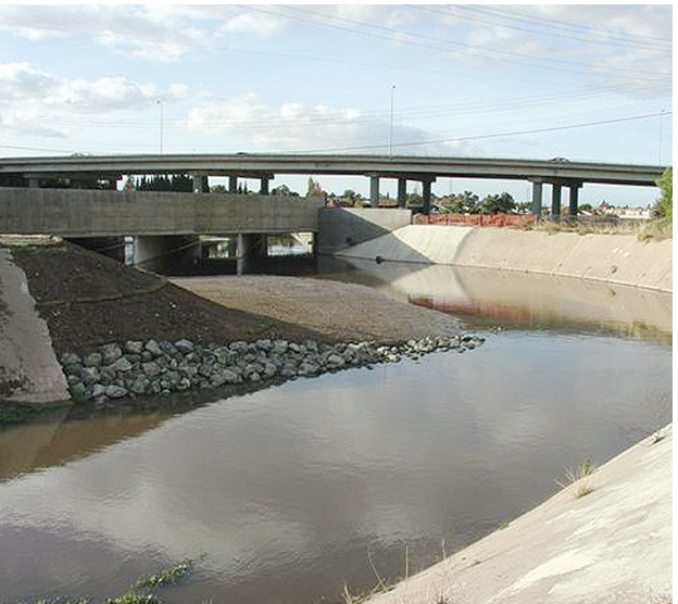
Berryessa Creek Levee looking north at Abel St. ridge.
