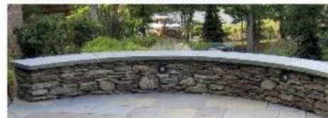
CURVED SEATWALL WITH STONE VENEER
