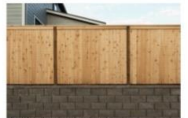
WOOD FENCE ON RETAINING WALL
