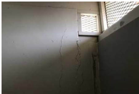
#65 FOOTHILL PARK, STRUCTURAL CRACK
