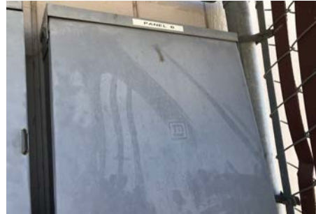
#14 RUSSELL MIDDLE RESTROOM, DISTRIBUTION PANEL, 208 Y, 120 V, 100 AMP
