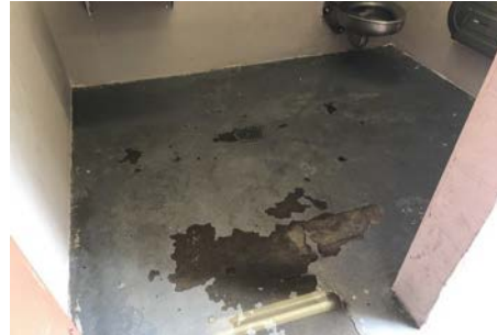
#62 PINEWOOD EPOXY FLOOR COATING DEGRADATION
