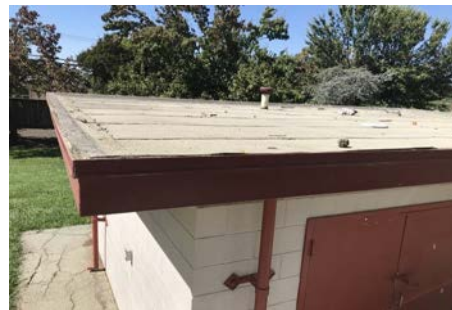
#16 CARDOZA ROOF, MODIFIED BITUMINOUS
