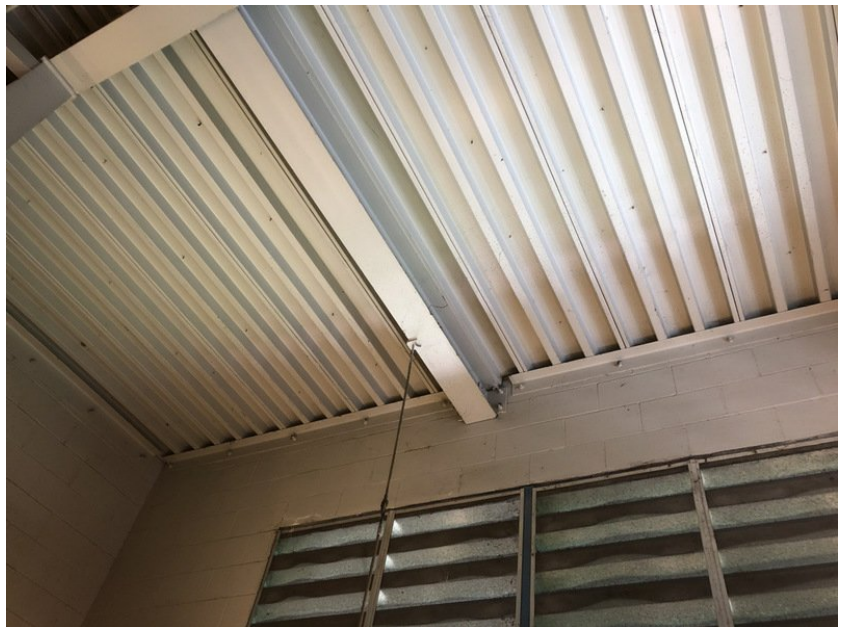
TYP wall to roof connection
