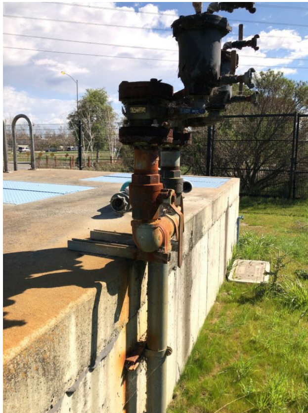
Corroded metal attachment
