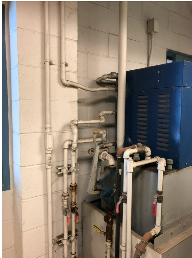
Piping on one side, piping attached to wall, flexible connection for 2 lines only (2 gray pipes coming out of slab), 4 red shutoff valves
