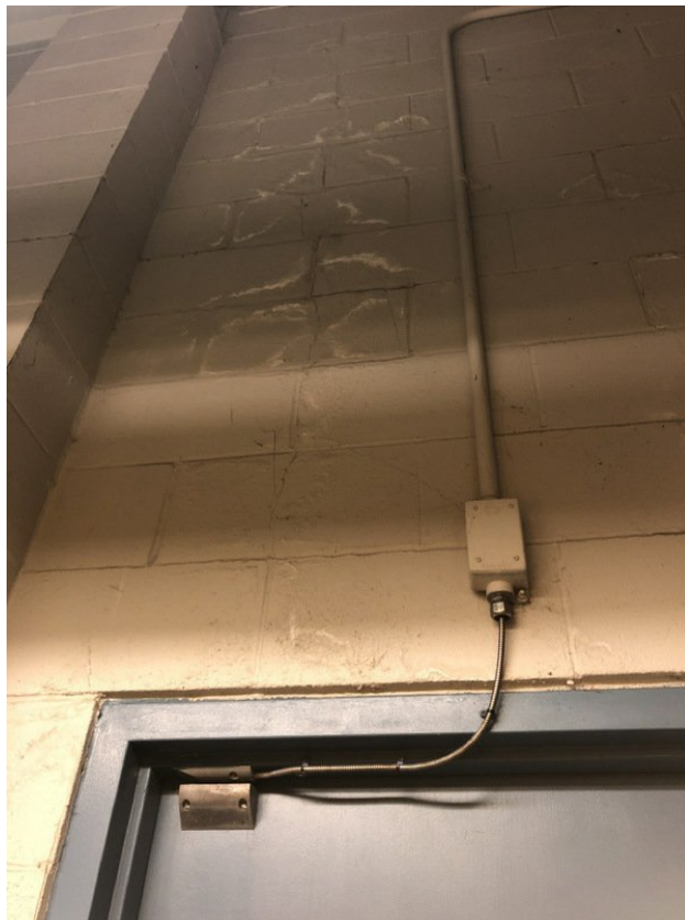
Cracks inside, right side of building
