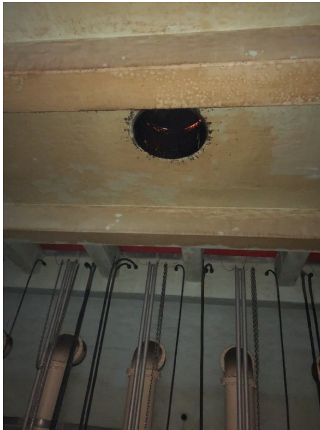
Penetration on opposite side of grit chamber
