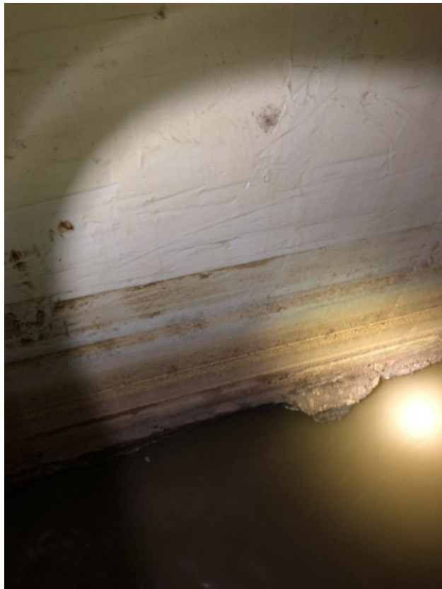
Dirt on steel not corrosion
