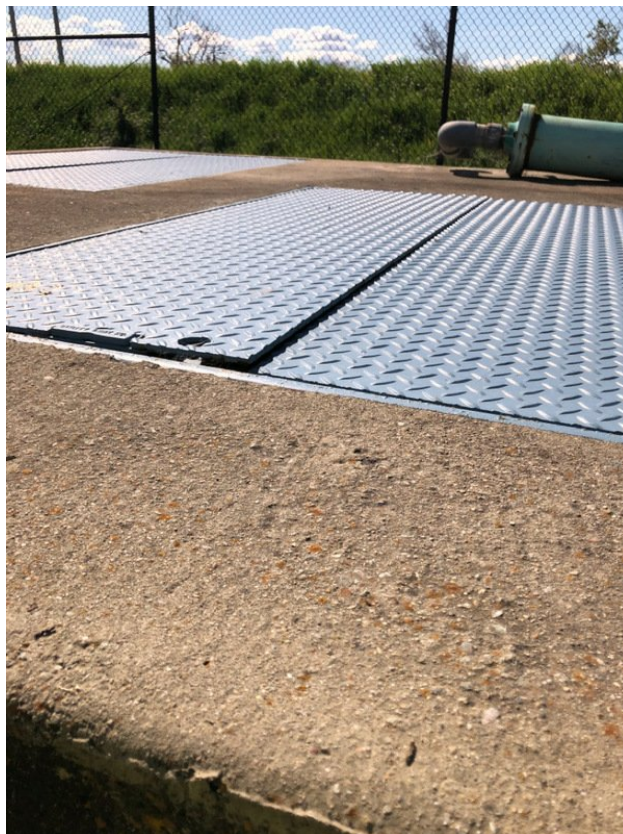
Spalling concrete
