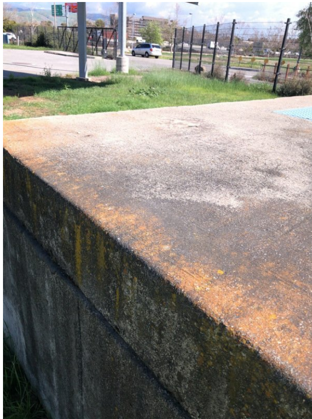
Exposed aggregates, sim to 2
