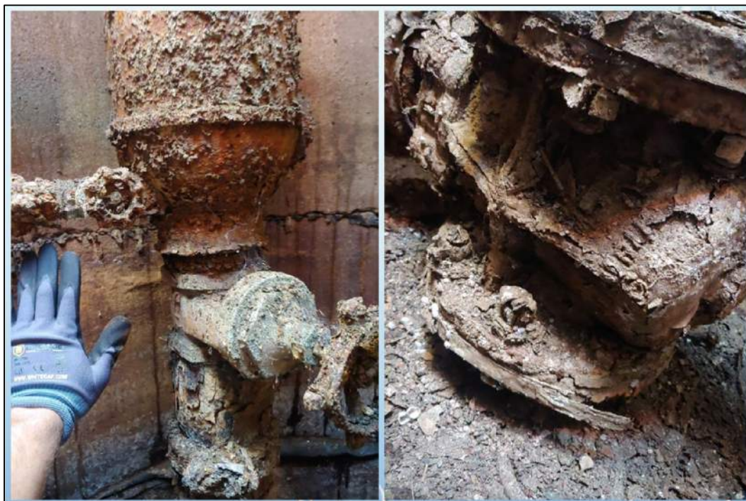
Figure 9: Corroded Air Release Valve and Blind Flange
