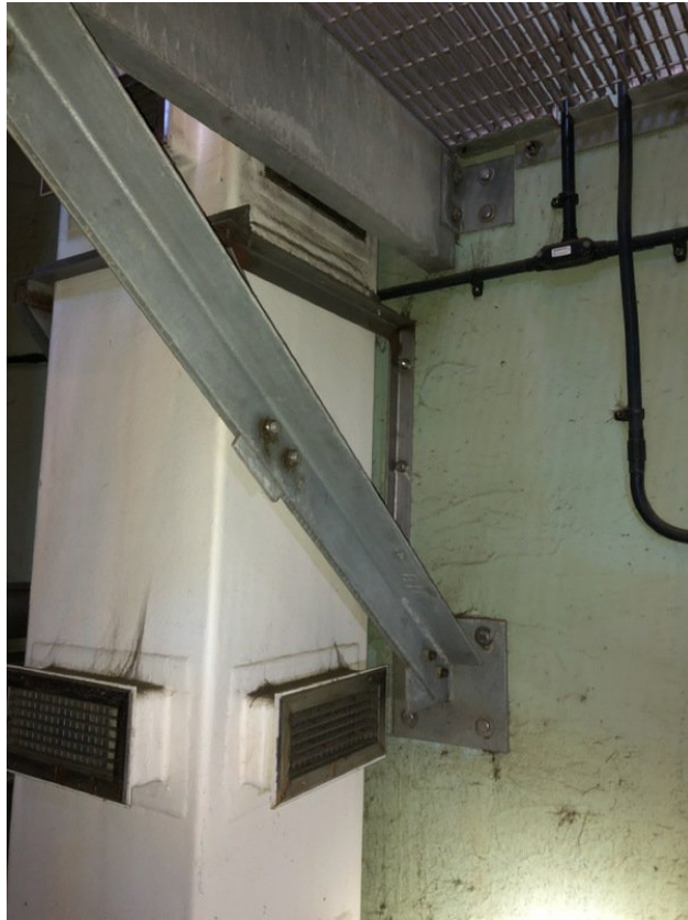
Stair knee brace connection
