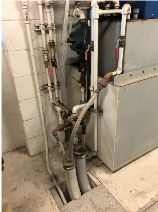
Piping on one side, piping attached to wall, flexible connection for 2 lines only (2 gray pipes coming out of slab), 4 red shutoff valves
