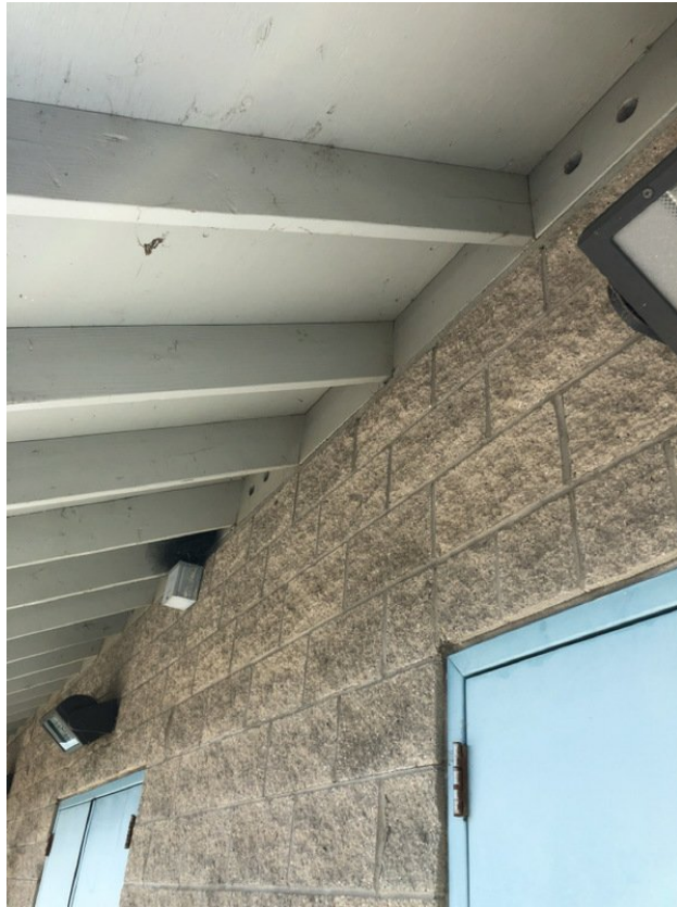
Connection to roof, from outside, vertical blocking different than what is shown on drawing
