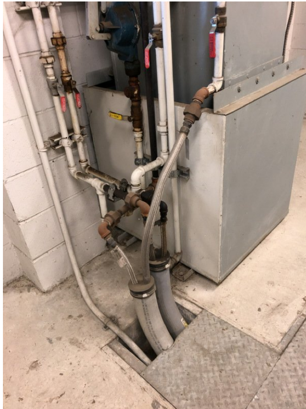
Connects to day tank, flexible coupling here
