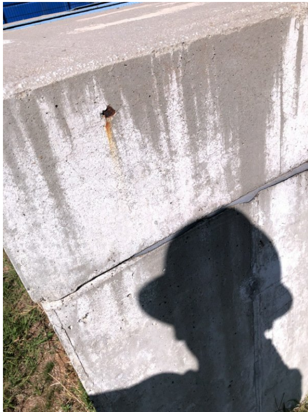
Exposed rebar
