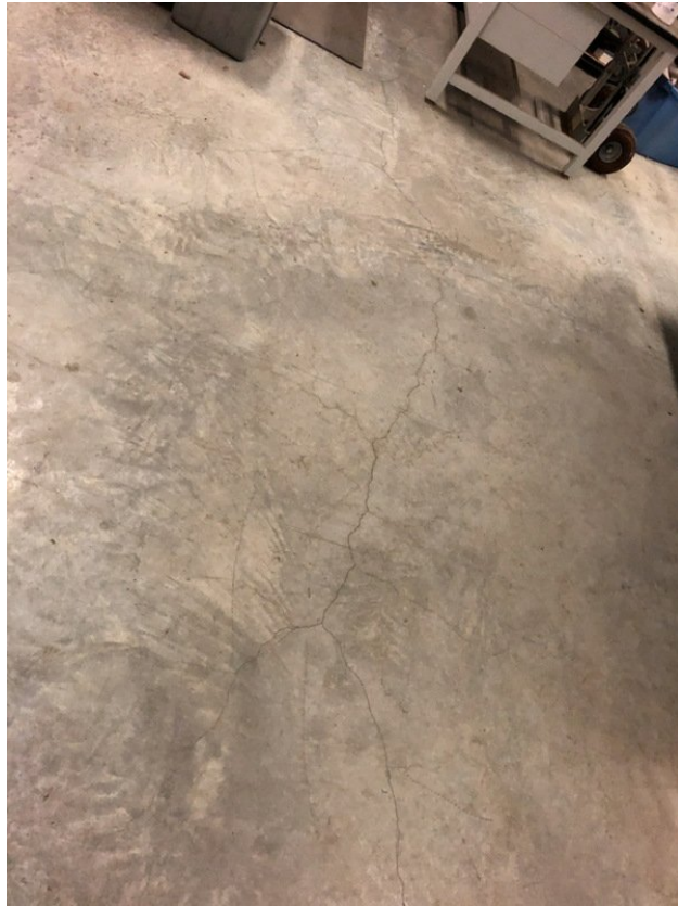
Cracks in slab, inside view, when it rains, water propagation follows cracks (water may have come up through cracks)
