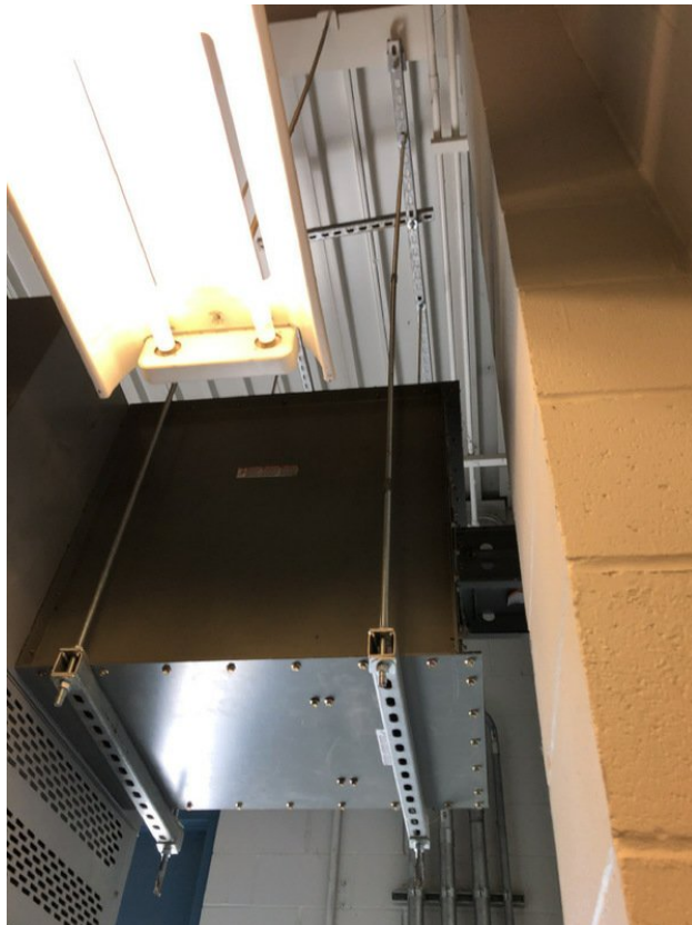
Electrical equipment supposedly anchored, though not visible outside
