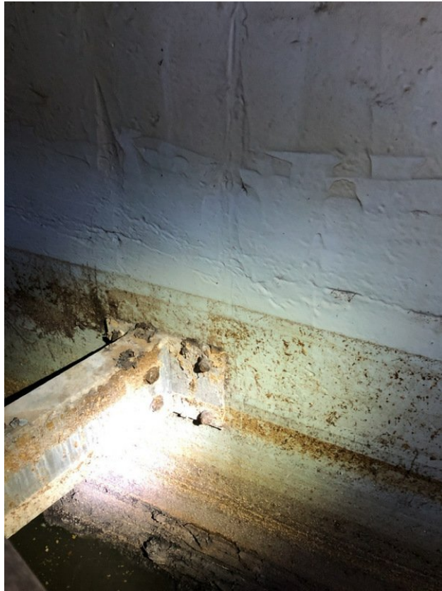
Dirt on steel not corrosion
