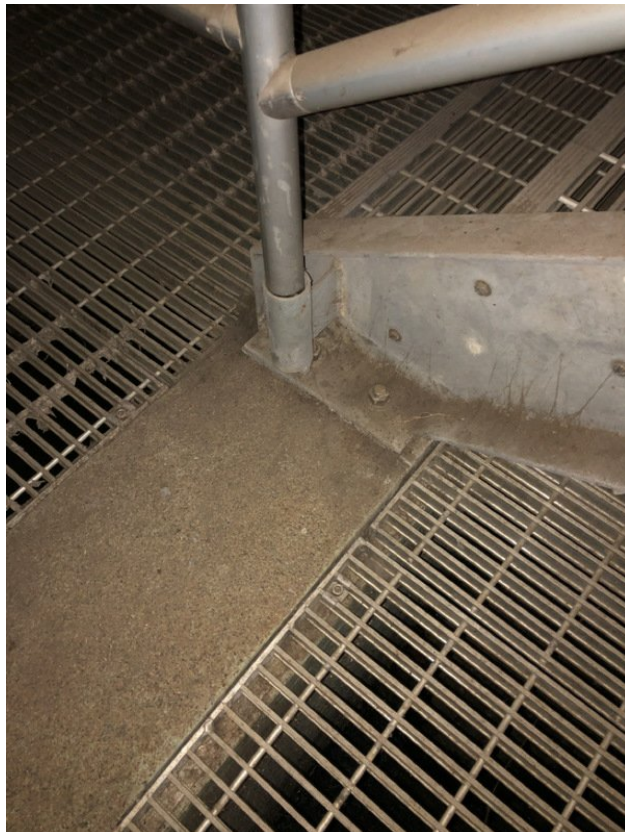
Stair knee brace connection
