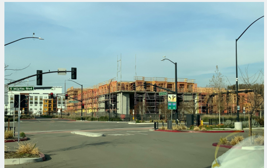
Lantana , 1675 S. Milpitas Blvd., a 5-story, 216-unit multifamily residential with commercial development. Photo shows the concrete work completed and wood framing in progress for the residential units on the 4th floor. Interior walls are completed in the garage.
